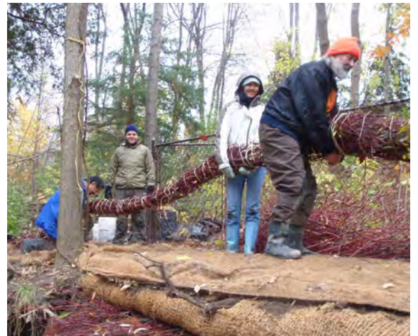
Building a fascine with volunteers as part of a bioengineering project in my past work at Rideau Valley Conservation Authority.
